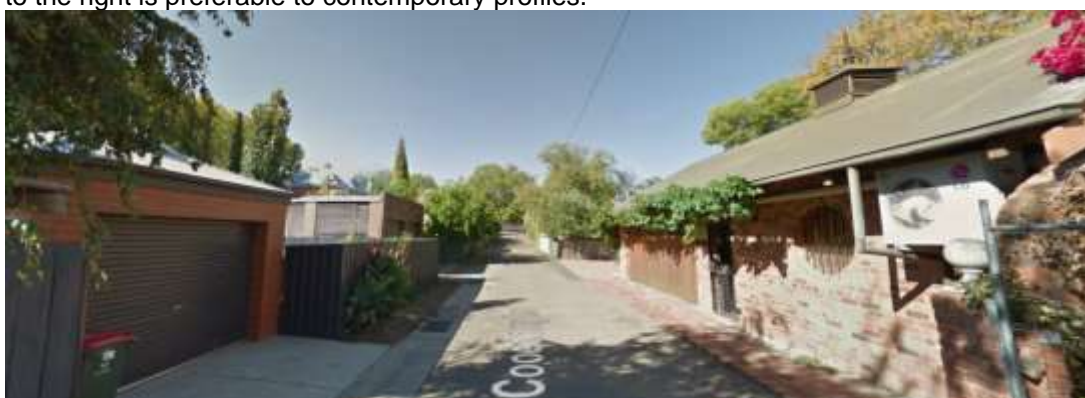
Figure 10 View looking east indicating varied setbacks, substantial brick structures and varied built forms.
