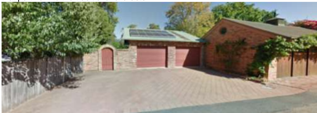
Figure 11 No 7 provides a vehicle manoeuvring space off the Lane with high brick walls and garage with gabled roof. The adjoining property No.9 builds closer to the Lane boundary and offers a brick garage structure with timber doors to the Lane and traditional gabled roof facing the Lane.
