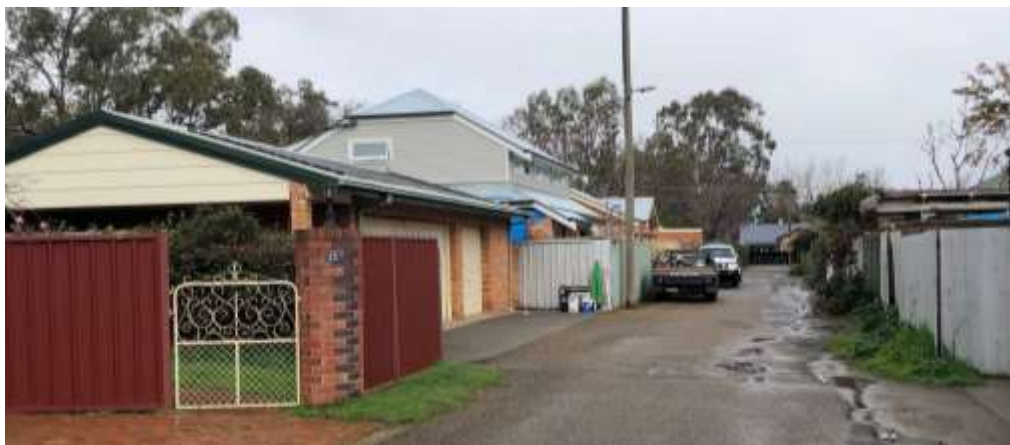
Figure 14 View to the west of the new development at No.17.
