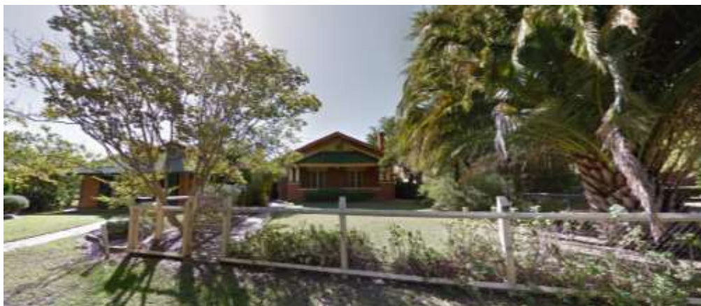
Figure 20 No. 15 is a contemporary brick house with dormer elements in the hipped steel roof with a bulk, form and materials intended to be sympathetic with the character while No. 13 is a typical brick bungalow with symmetrical plan, gabled roofs and elaborate details to the gables and verandah.
