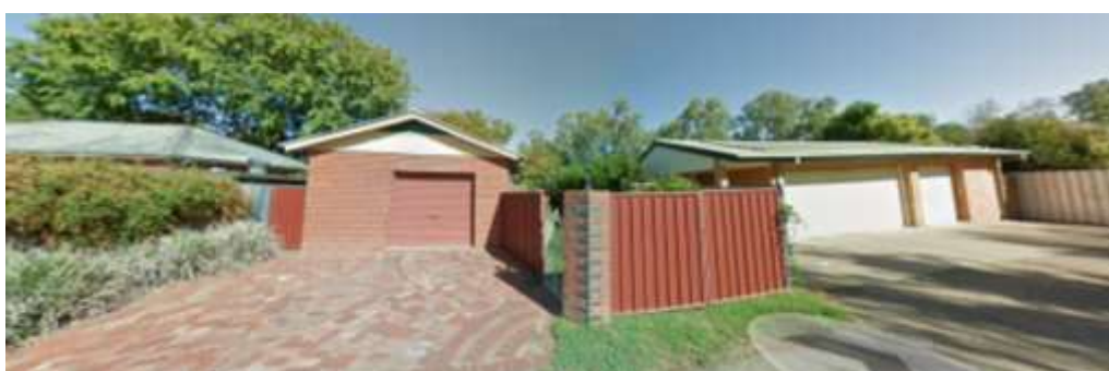
Figure 12 13 & 15 Wollundry Avenue provide vehicle setbacks to the Lane and two forms of brick garage. One displays a gable frontage with red brick walls and the larger uses the linear ridge with roof and two end gables.
