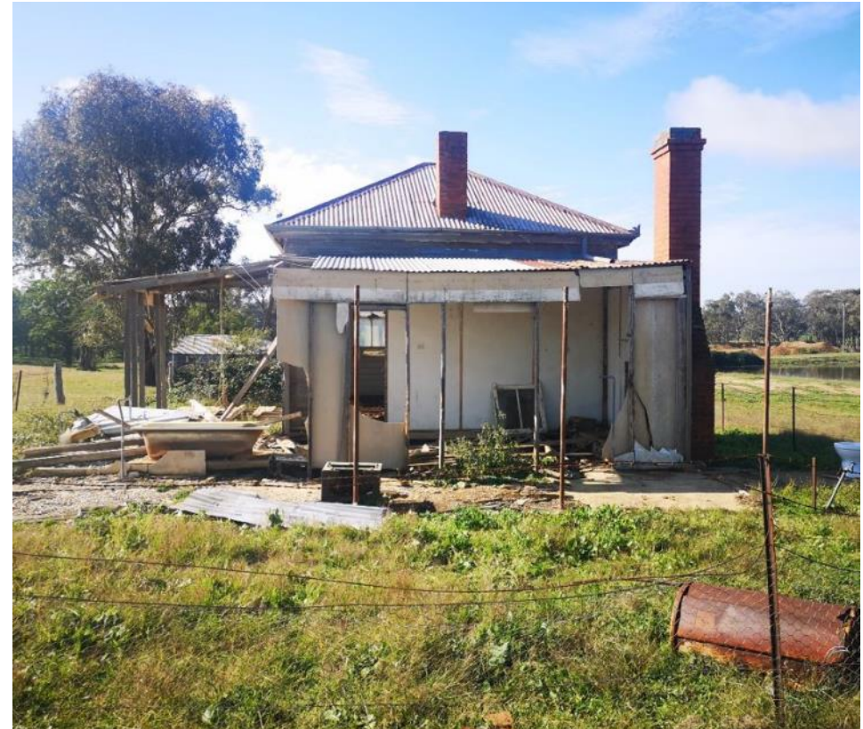
Figure 2-13 Derelict workers cottage – western elevation (Source: NGH, 2020)
