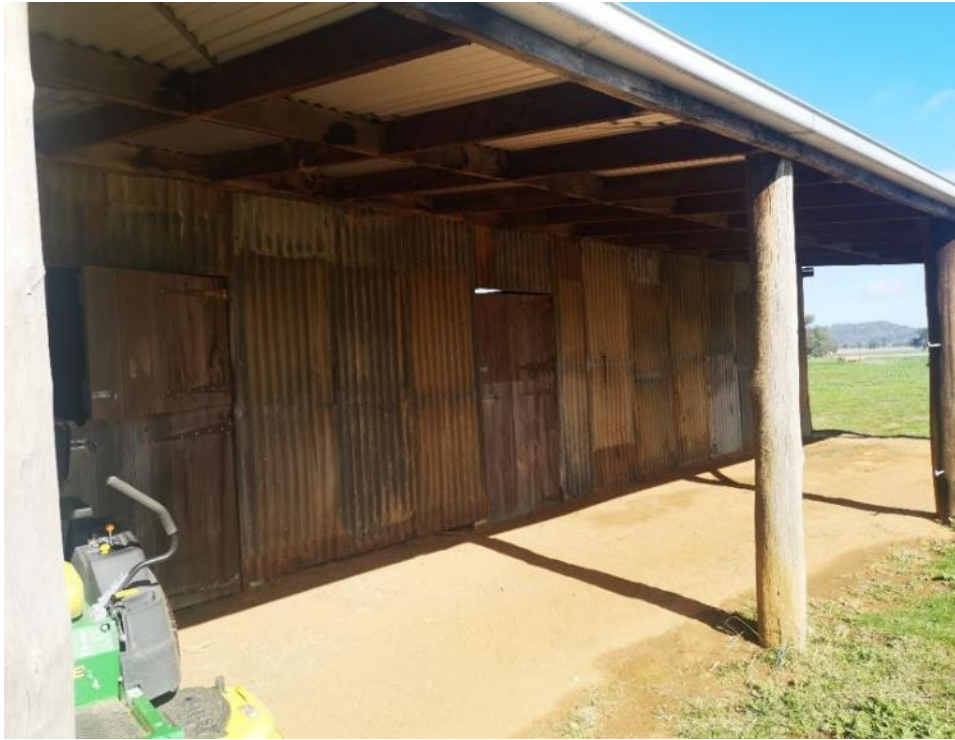
Figure 2-14 Former stables, currently used for storage (Source: NGH, 2020)
