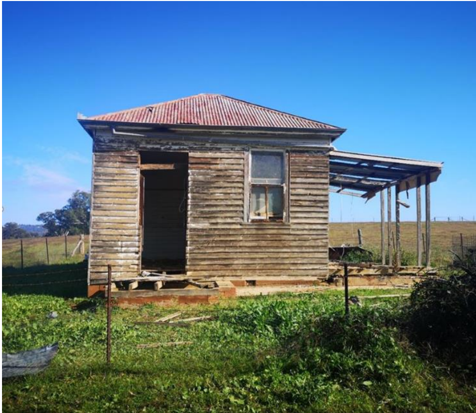
Figure 2-12 Derelict workers cottage – eastern elevation (Source: NGH, 2020)
