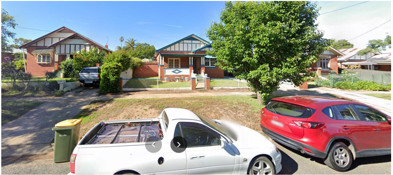
Figure 5 Nos. 26, 28 and 30 Gormly Avenue located to the rear of the subject site
