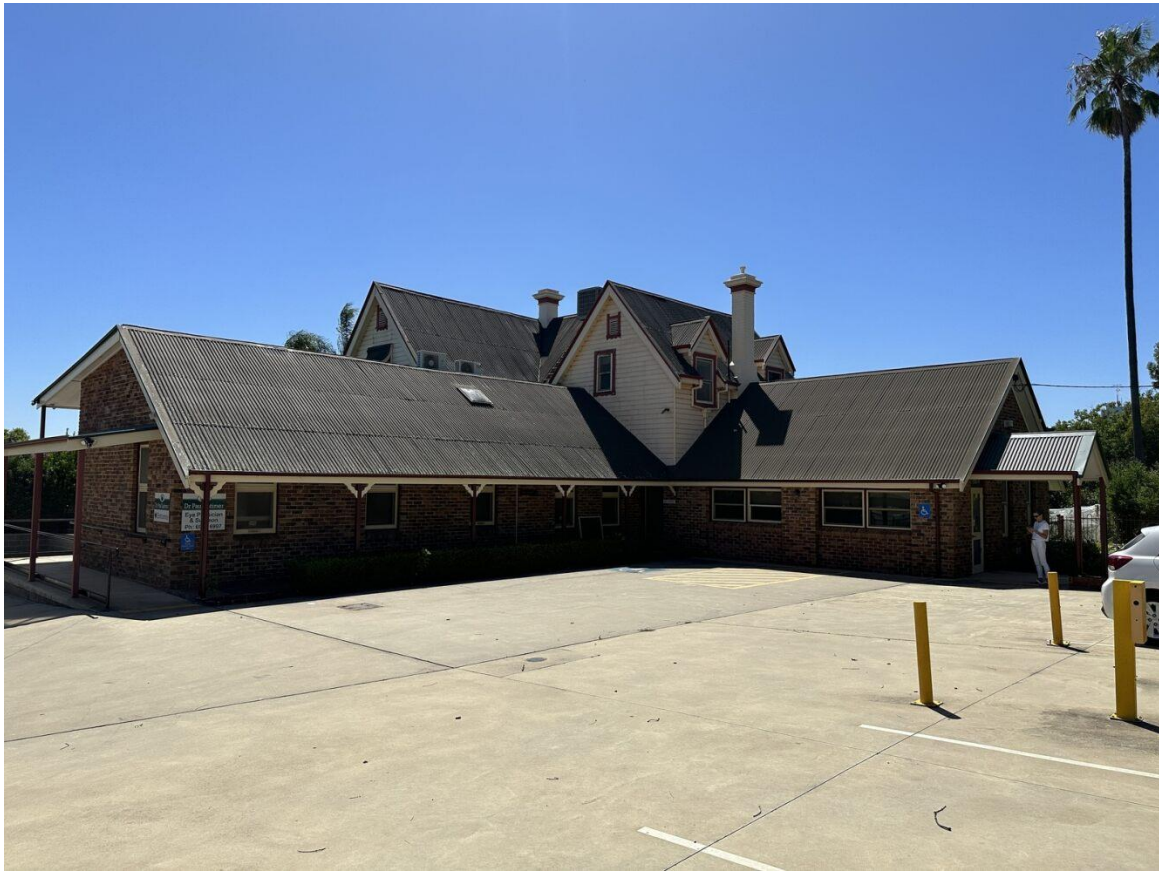
Figure 2 View of the subject site
