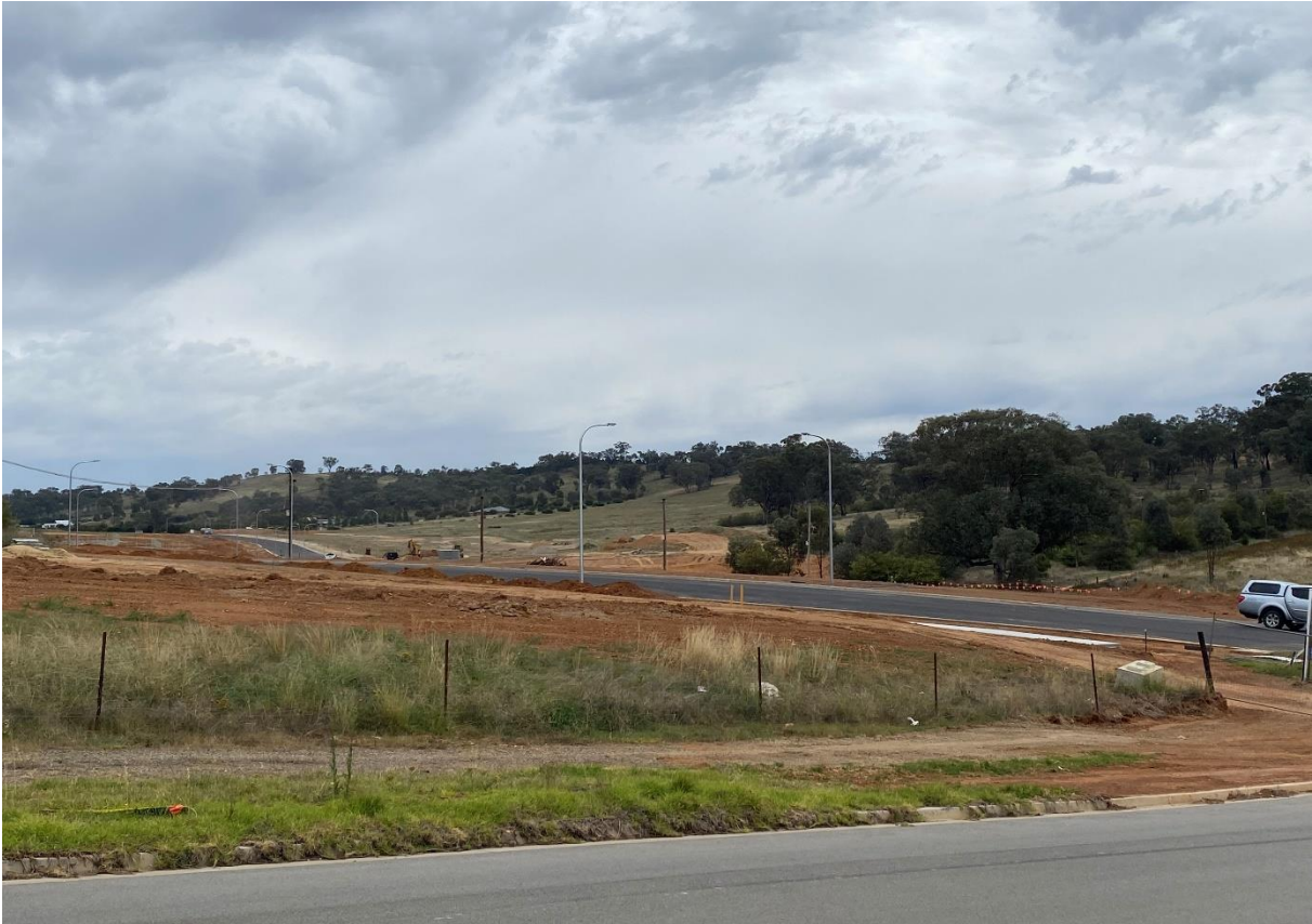
Photo of Deakin Avenue extension (24 January 2024)
