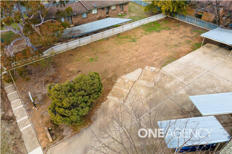
Image 5: Shows concrete pad for 2 carports that were demolished from fire. Image reference: One Agency real estate photos 2024.
