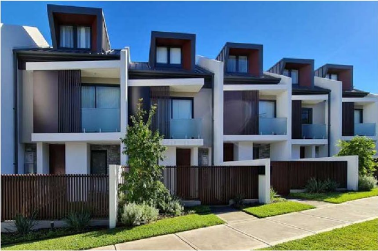
Figure 11 Example of townhouses (23 Stuart Street, Concord West)
