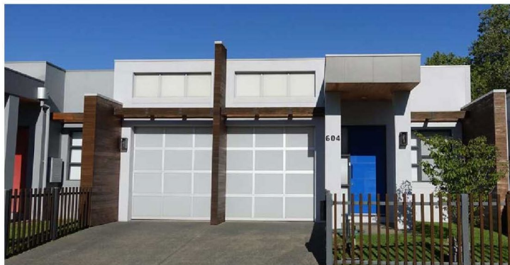
Figure 5 Example of semi-detached dwelling (604 Olive Street, Albury)
