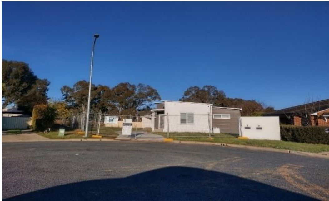
Figure 4: Site Photos Bowen Place
