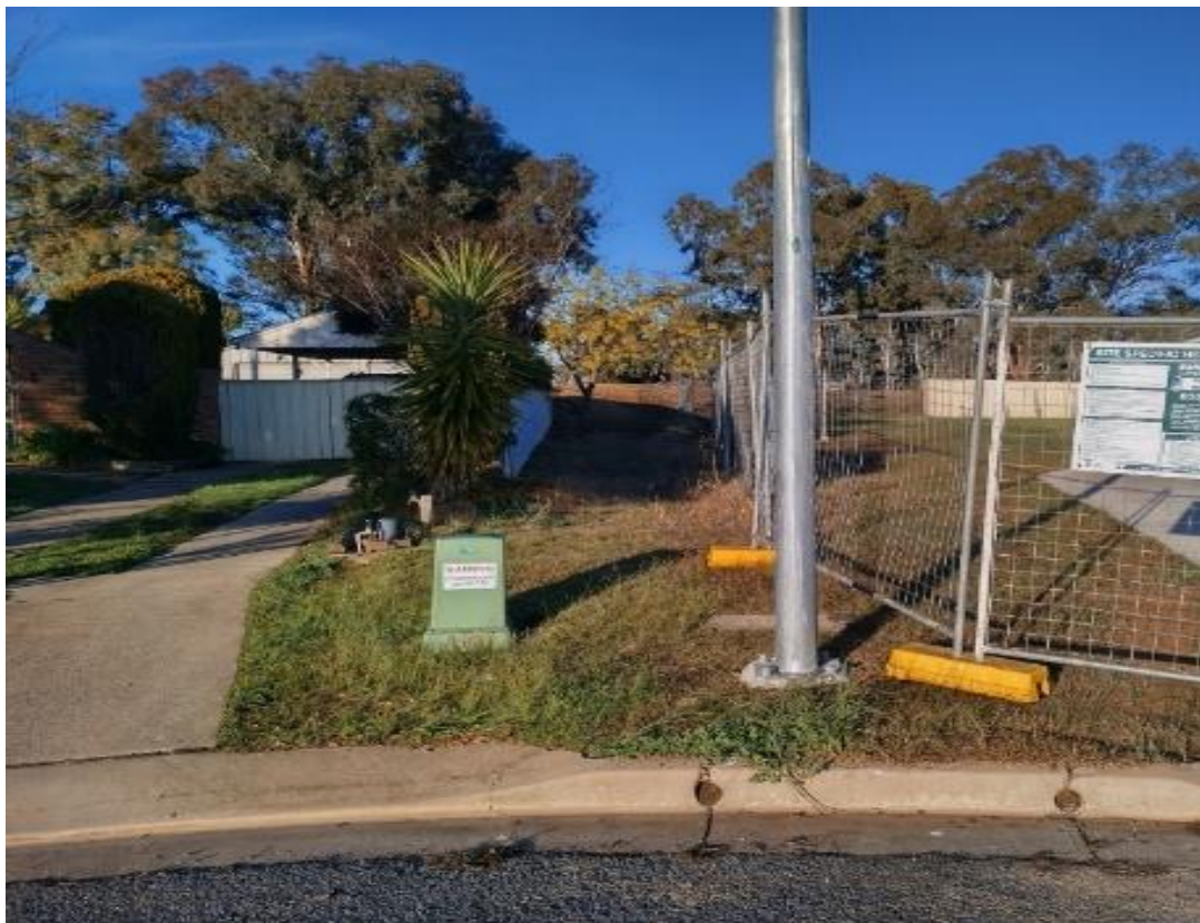
Figure 5: Site Photos Bowen Place
