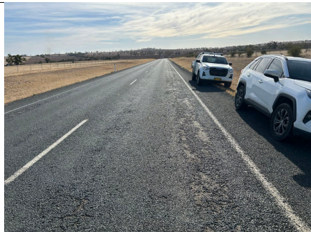
Stripping of sprayed seal, isolated areas between Olympic Highway and Dorset Drive
