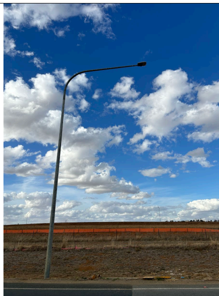
Lamp poles rotated off alignment after major storm. Essential Energy maintained
