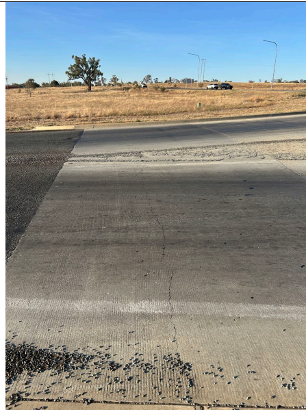
Minor concrete slab cracking in a slab at Byrnes road roundabout departure
