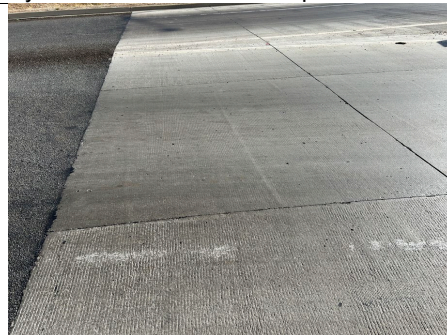
Worn texture in heavily trafficked sections of SFRC roundabout at Dorset Drive
