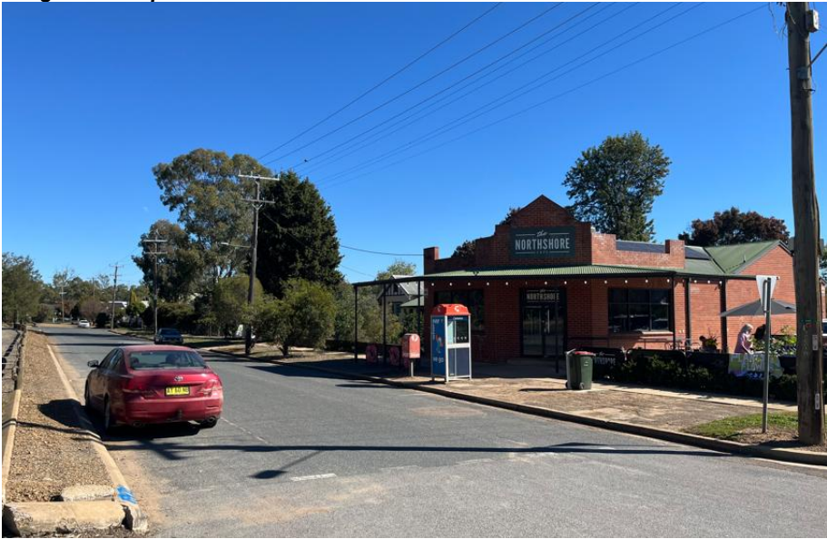
Image 3 - Hampden Avenue Service Road
