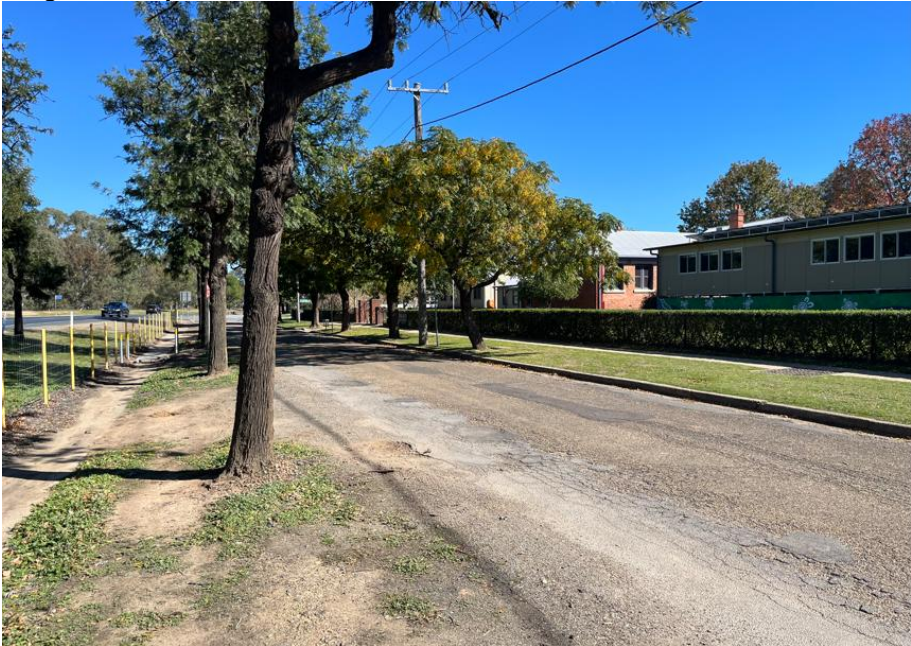
Image 2 - Hampden Avenue Service Road
