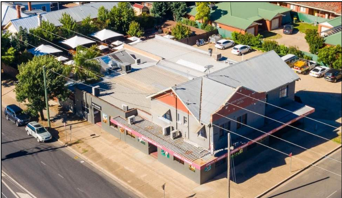
Figure 17: Historical Photo – 2020 - Kincaid/Beckwith St frontage (Source: Client Drone Image 2023)
