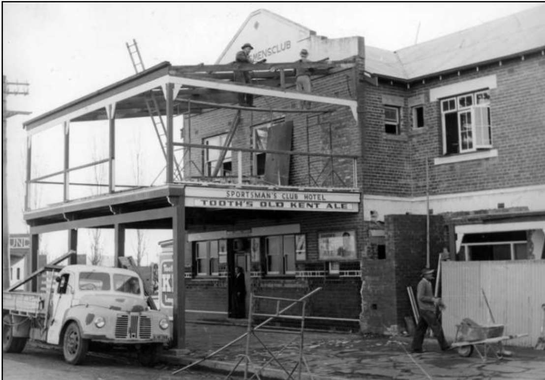
Figure 13: Historical Photo – 1965 – Post-supported verandah removal (Source: CSU Archives 2023)
