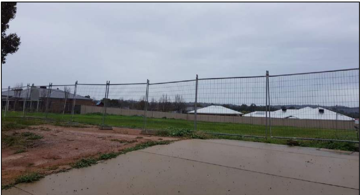
Figure 11: Existing Site Photo – View from Gregadoo Road (Source: SP 2021)
